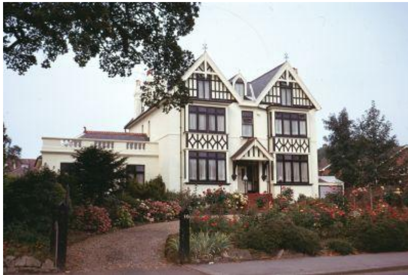
Fig. 7. Ten Bycullah Road: a good example of a large house on this estate.
